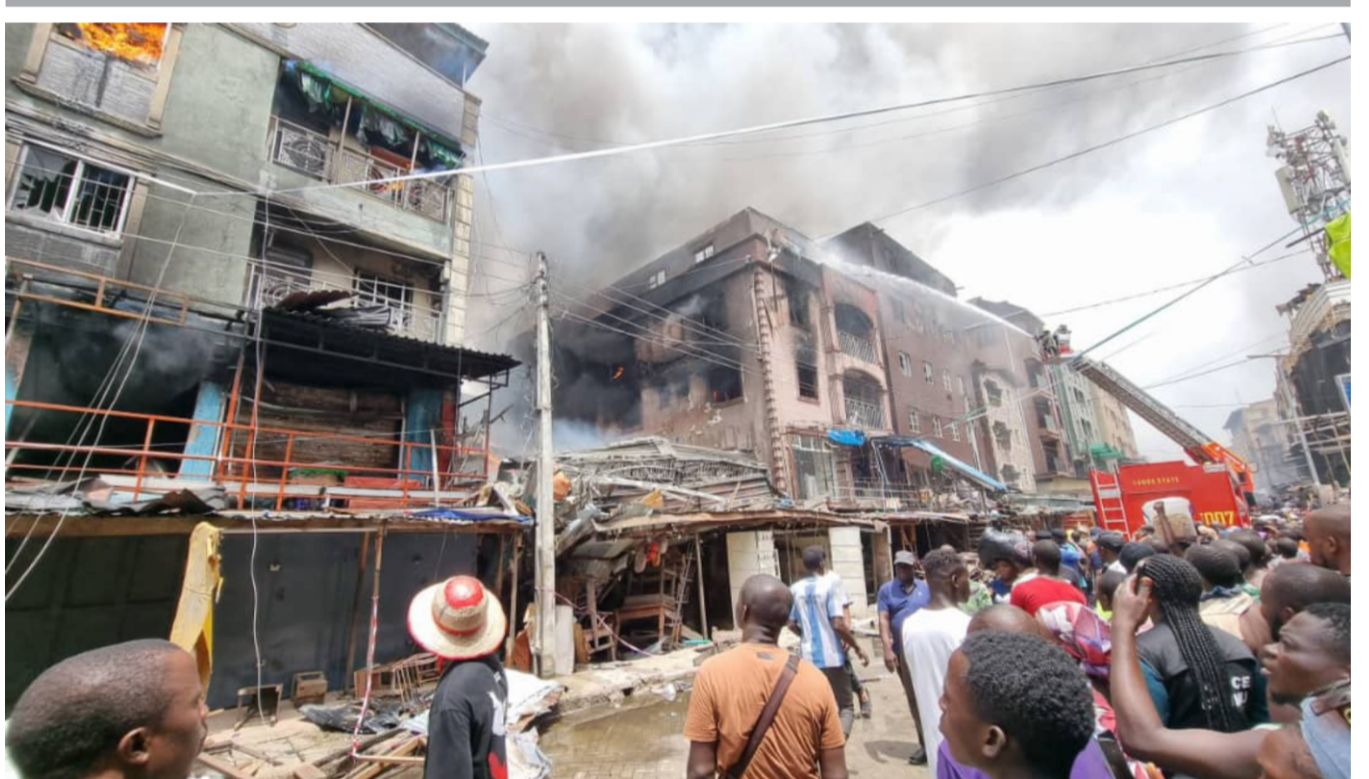
Fire outbreak burns four buildings at Docemo Street, Idumota in Lagos. Photo: AKINOLA ARIYO
