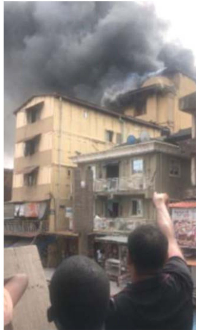
The affected building
